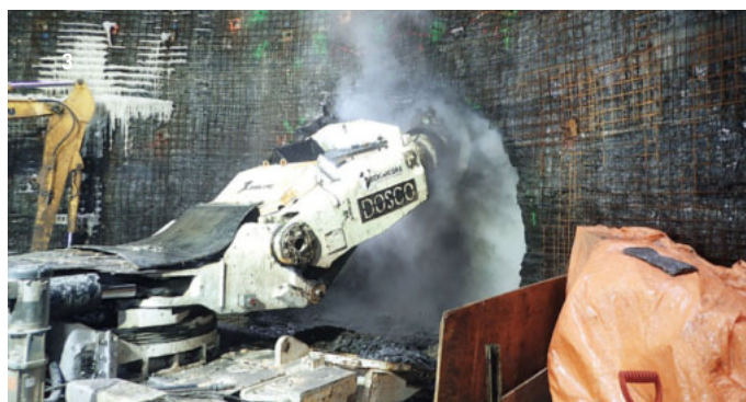
1 Finished tunnel (Precast elements) 2 Mid-Halton TBM "Peggie" 3 Tunnel excavation with road header
